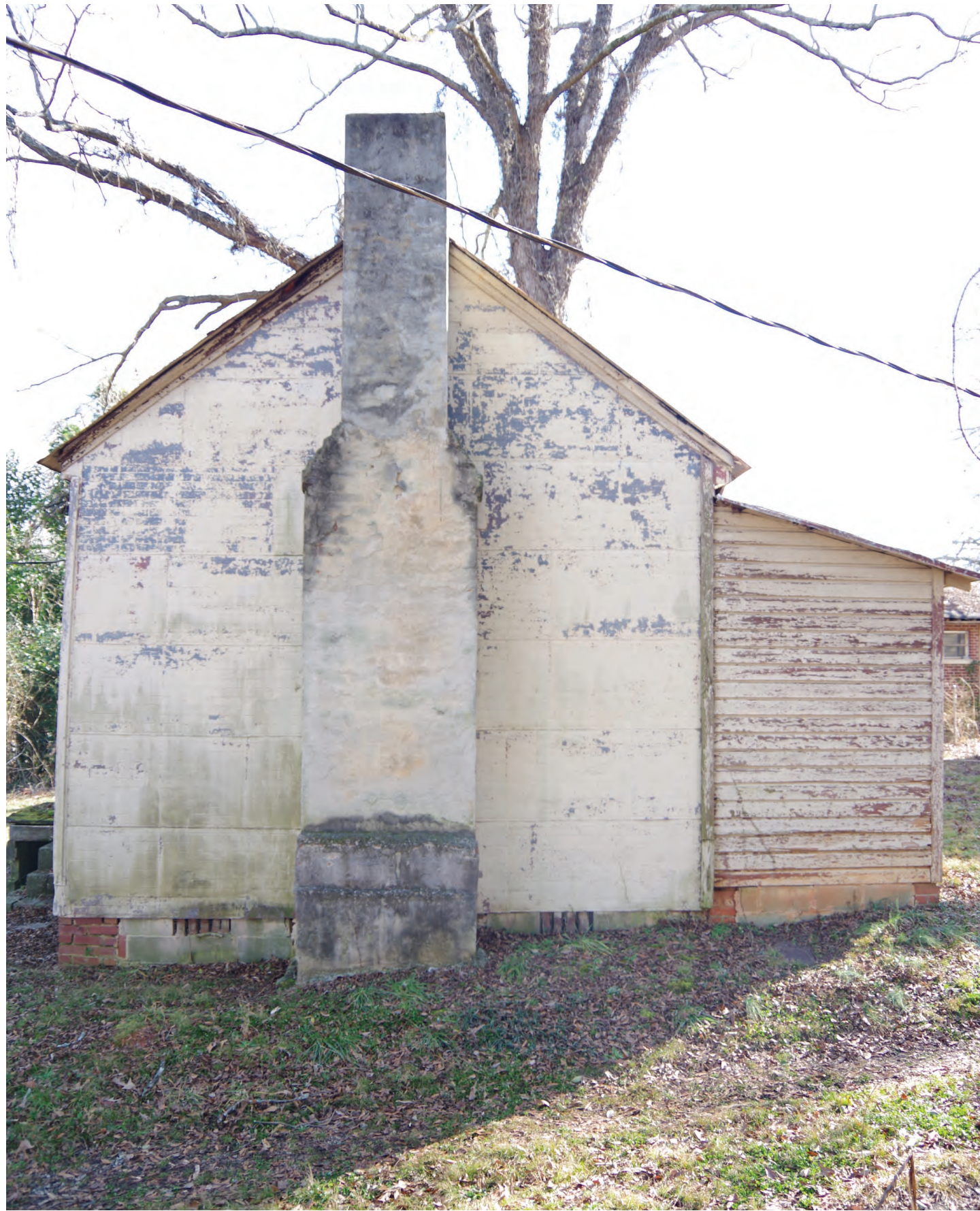
East elevation with addition on north end, brick pier foundation with CMU infill
