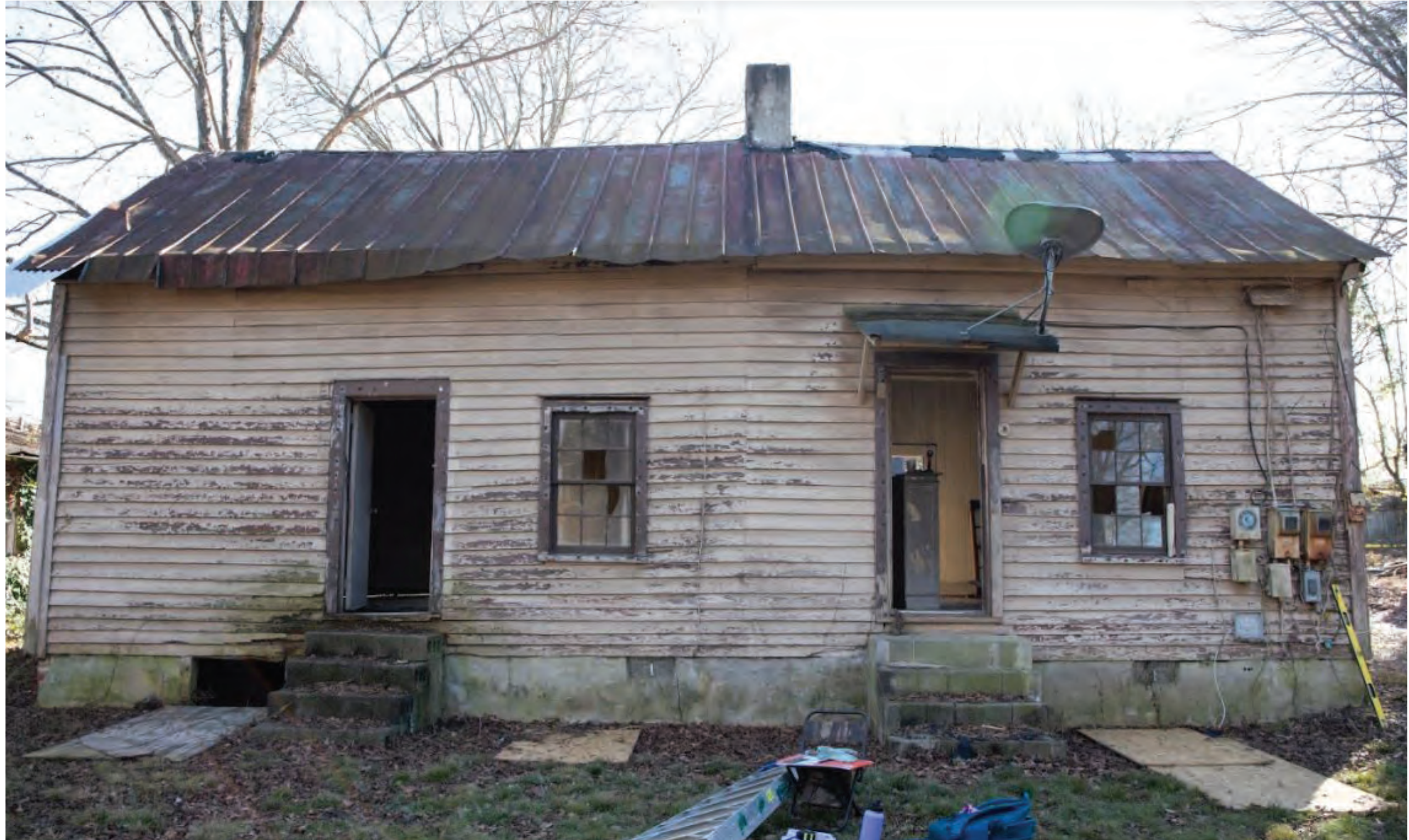
314 East Morris Street north elevation
