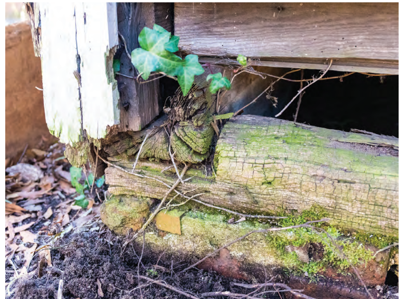
318 East Morris Street, northeast corner
