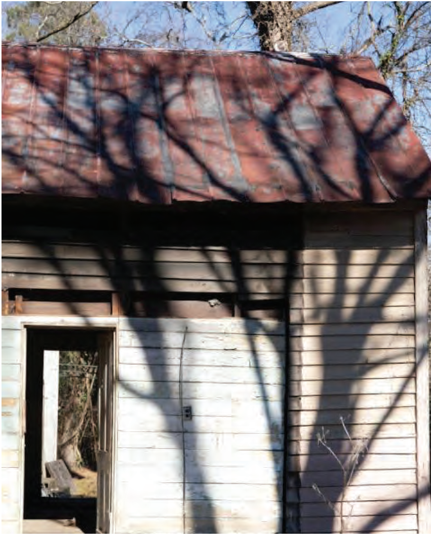
Metal seam roof and remnant of addition on the south facade
