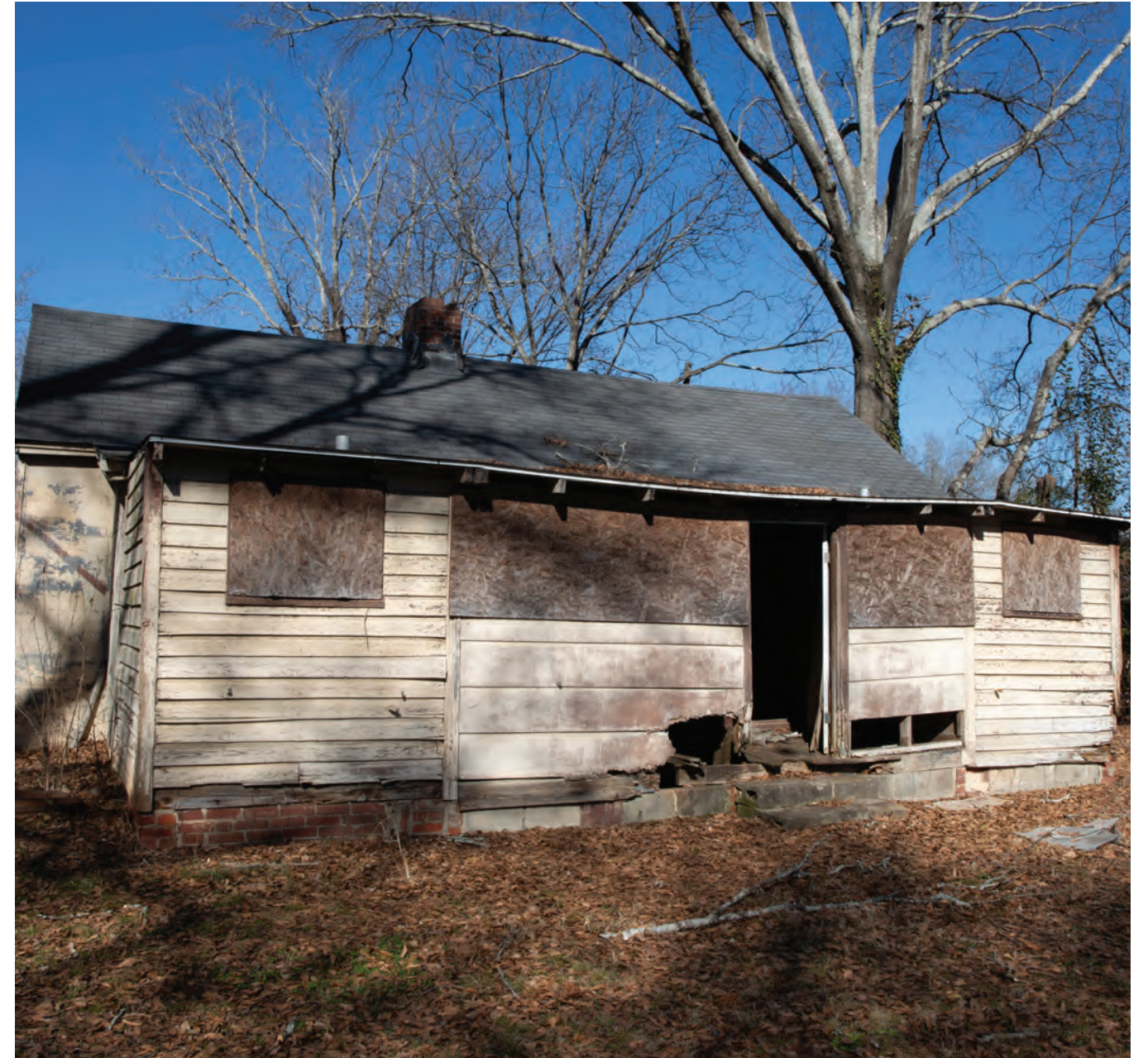
316 East Morris Street, south facade showing additions
