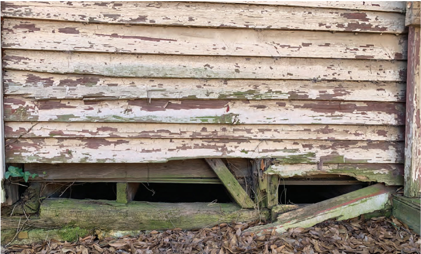
Northeast corner showing diagonal bracing resting on a hand-hewn sill plate
