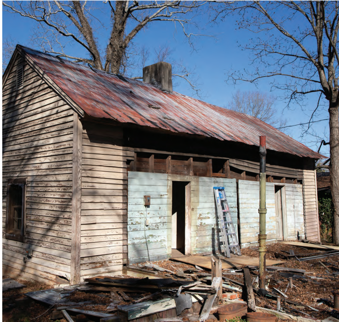
314 East Morris Street, south facade with porch remnants
