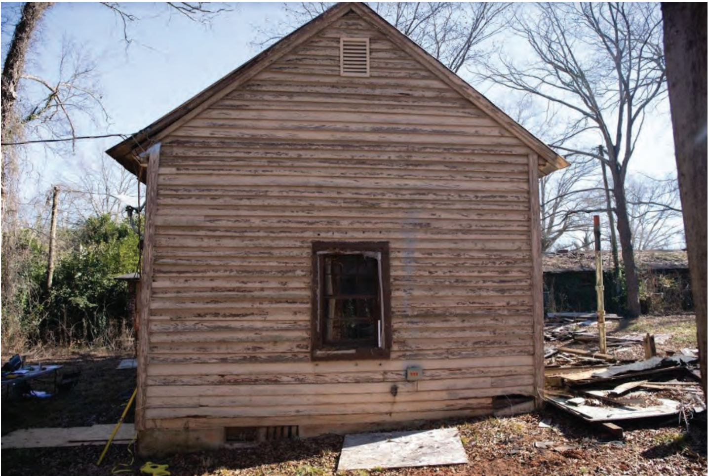
West facade showing sloping topography
