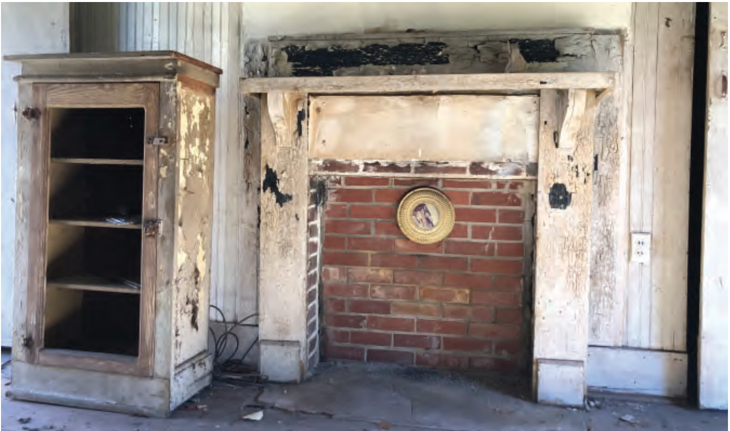
West room architectural piece and fireplace with extruded brick infill
