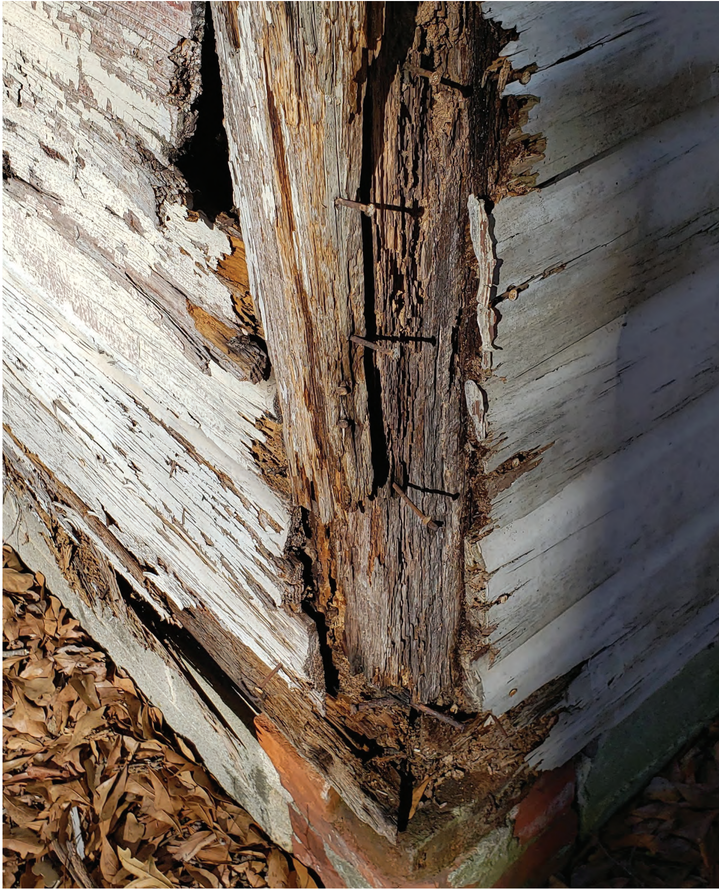
Corner post with wire nails and extruded brick pie foundation
