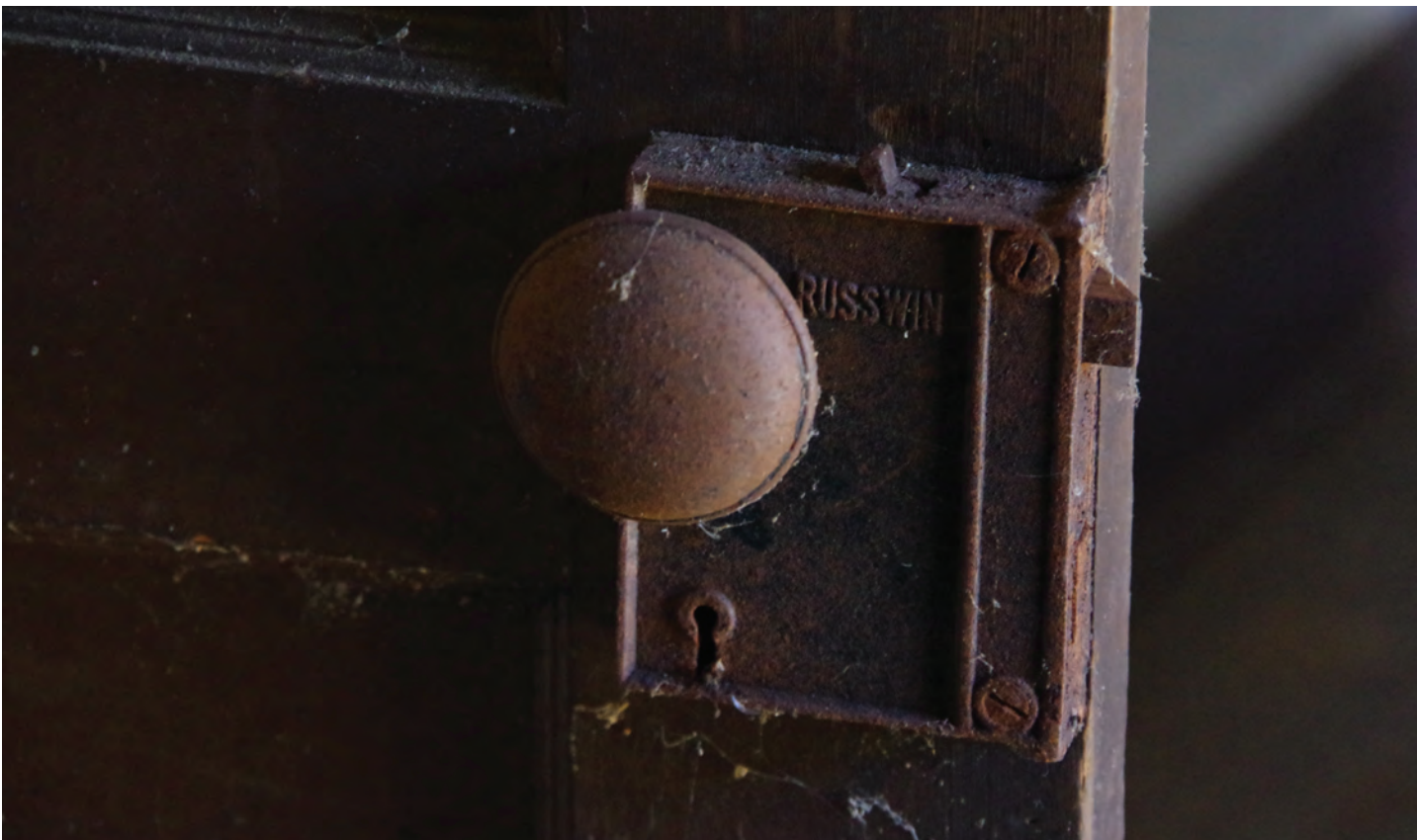
Door knob located on interior door
