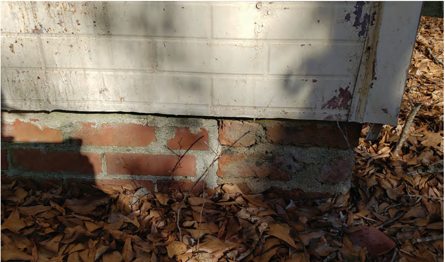
Brick pier foundation with extruded brick and portland cement mortar infill
