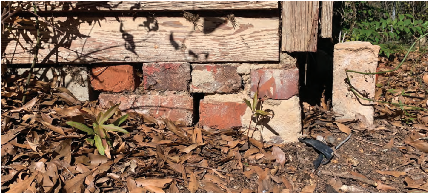
Brick pier foundation at southeast corner, utilizing both hand-molded and extruded bricks
