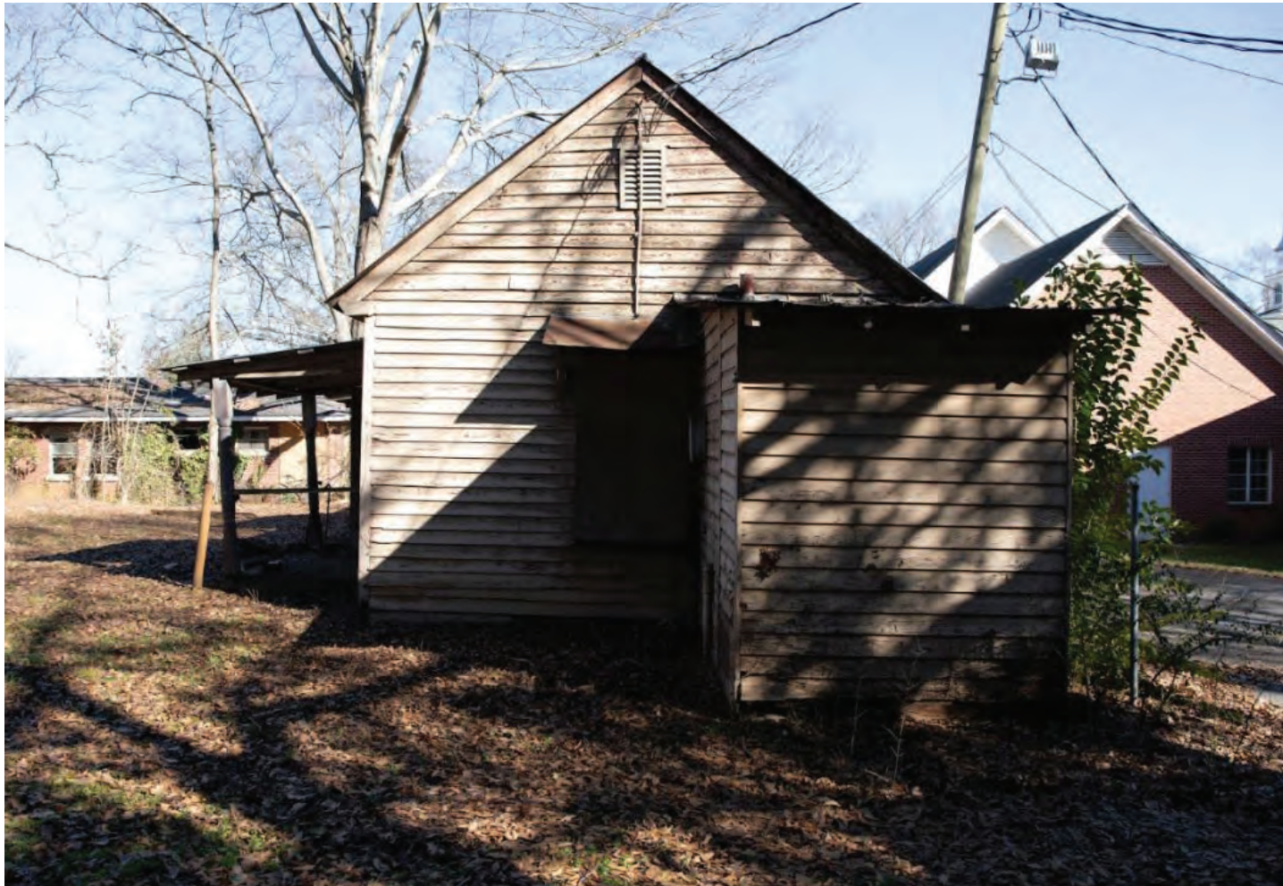
West elevation showing bathroom addition and porches
