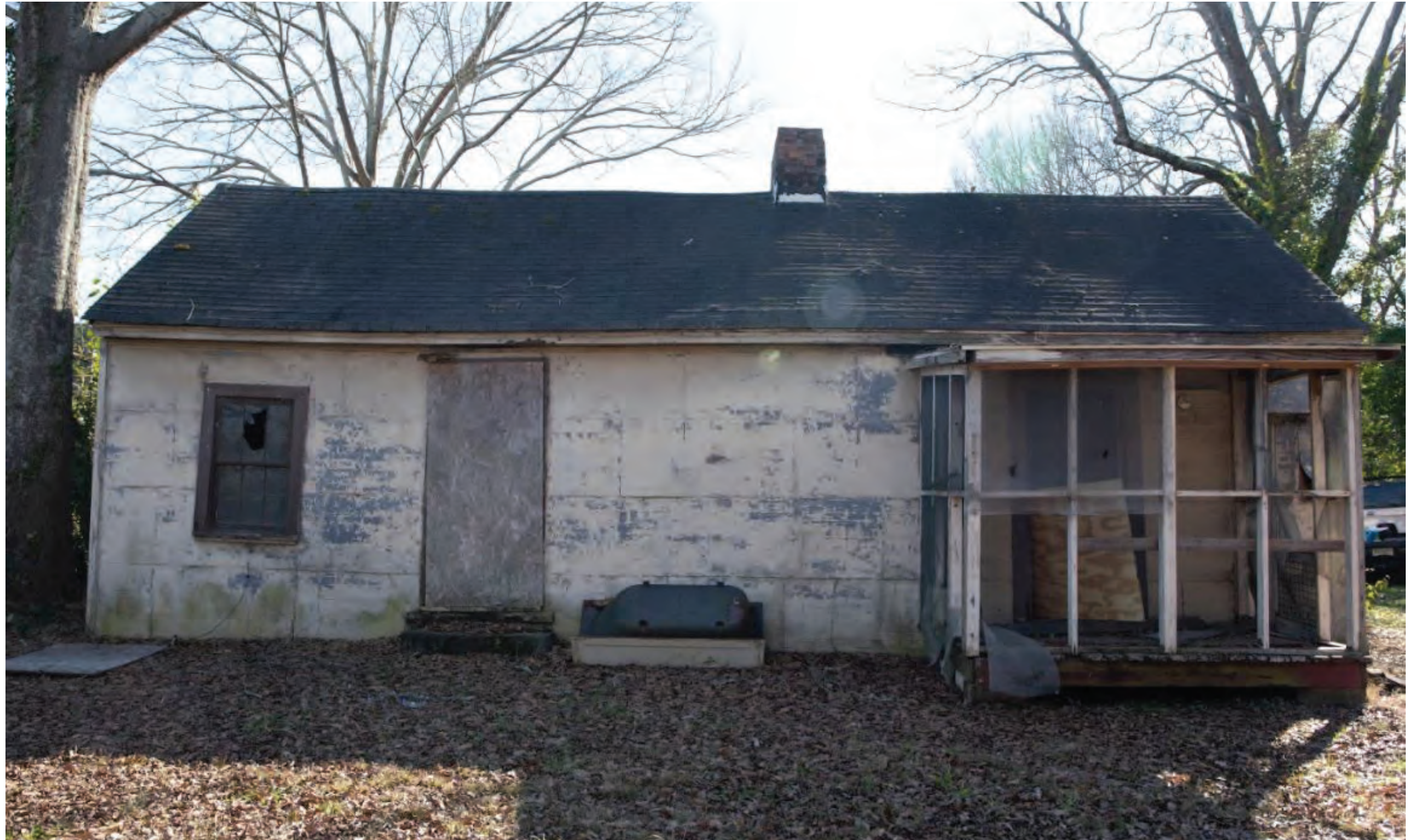
316 East Morris Street north elevation
