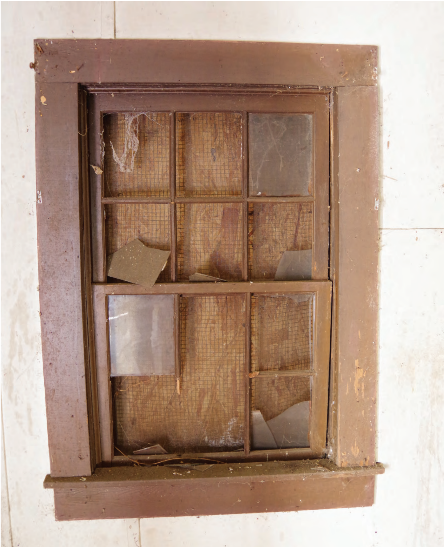
Interior window frame showing six-over-six light frame
