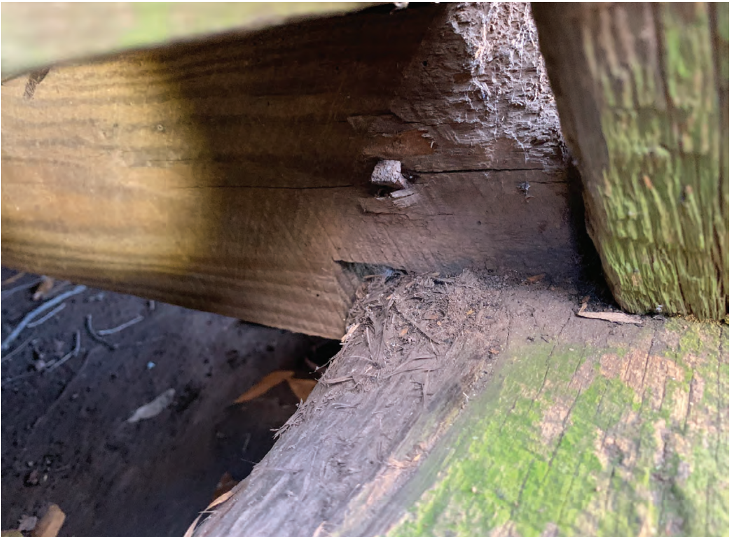
Floor joist at northeast corner showing circular saw marks and the reuse of materials such as a hand-wrought nail
