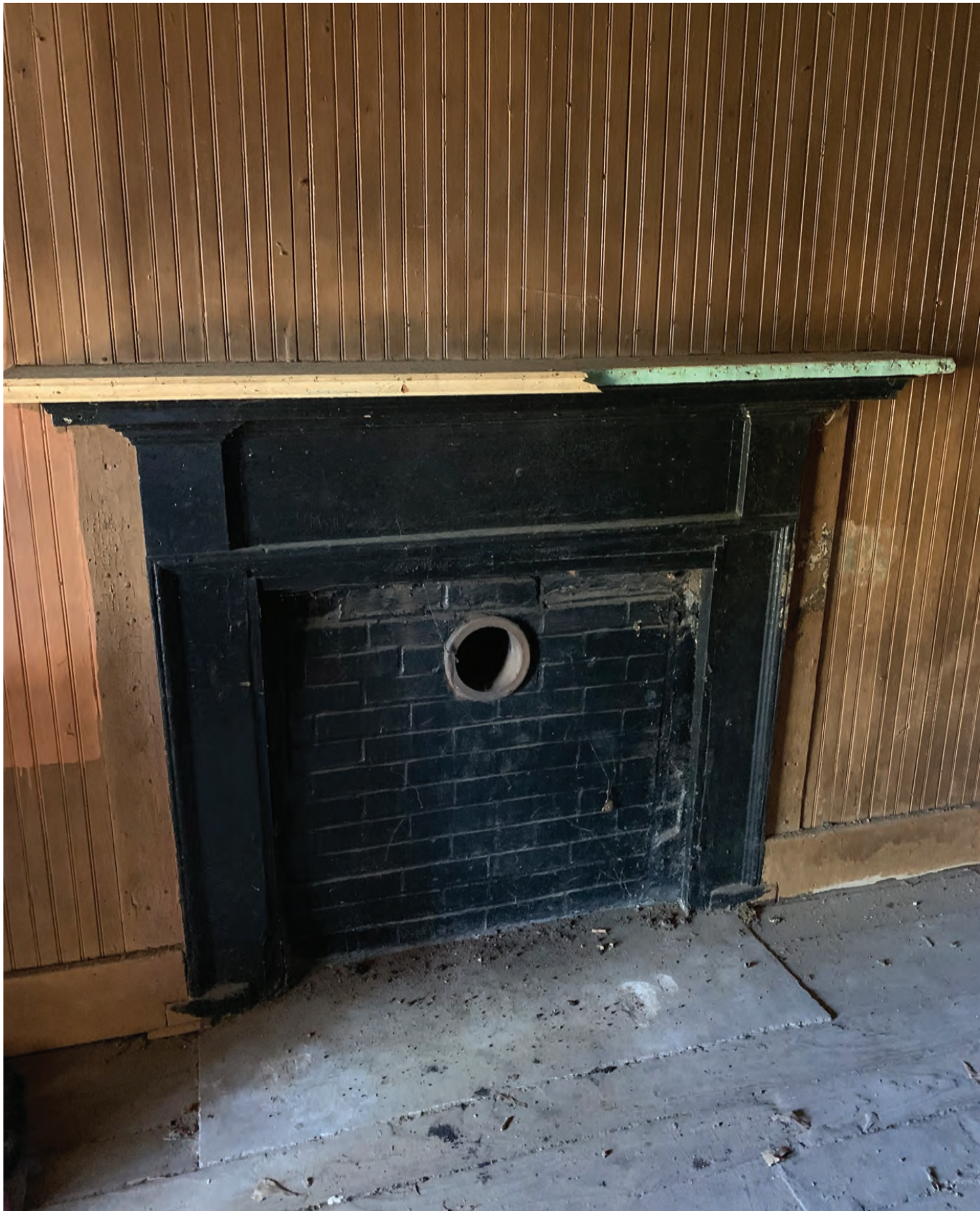
Mantel with brick infill and painted beadboard siding
