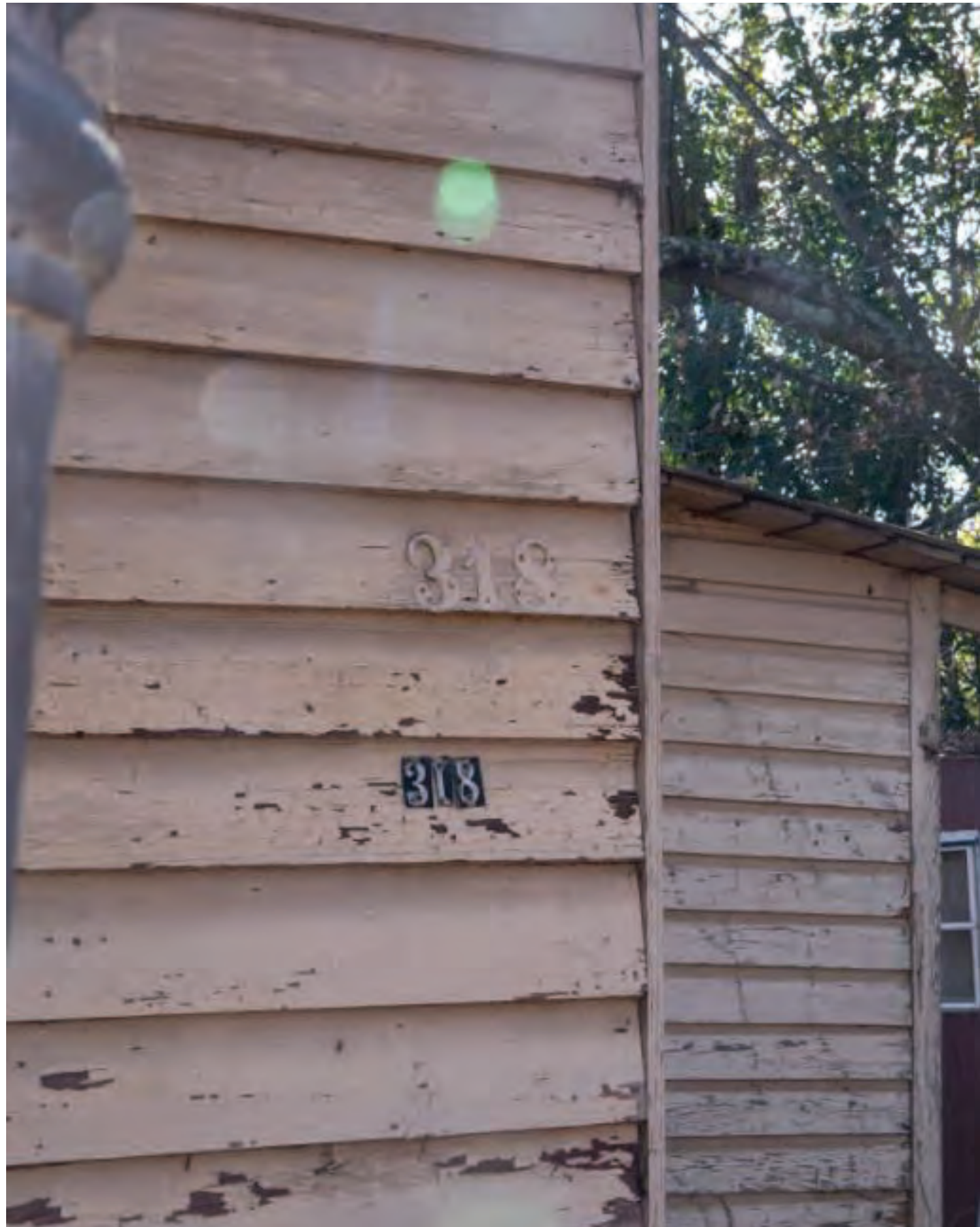
Various siding used on original building and bathroom addition
