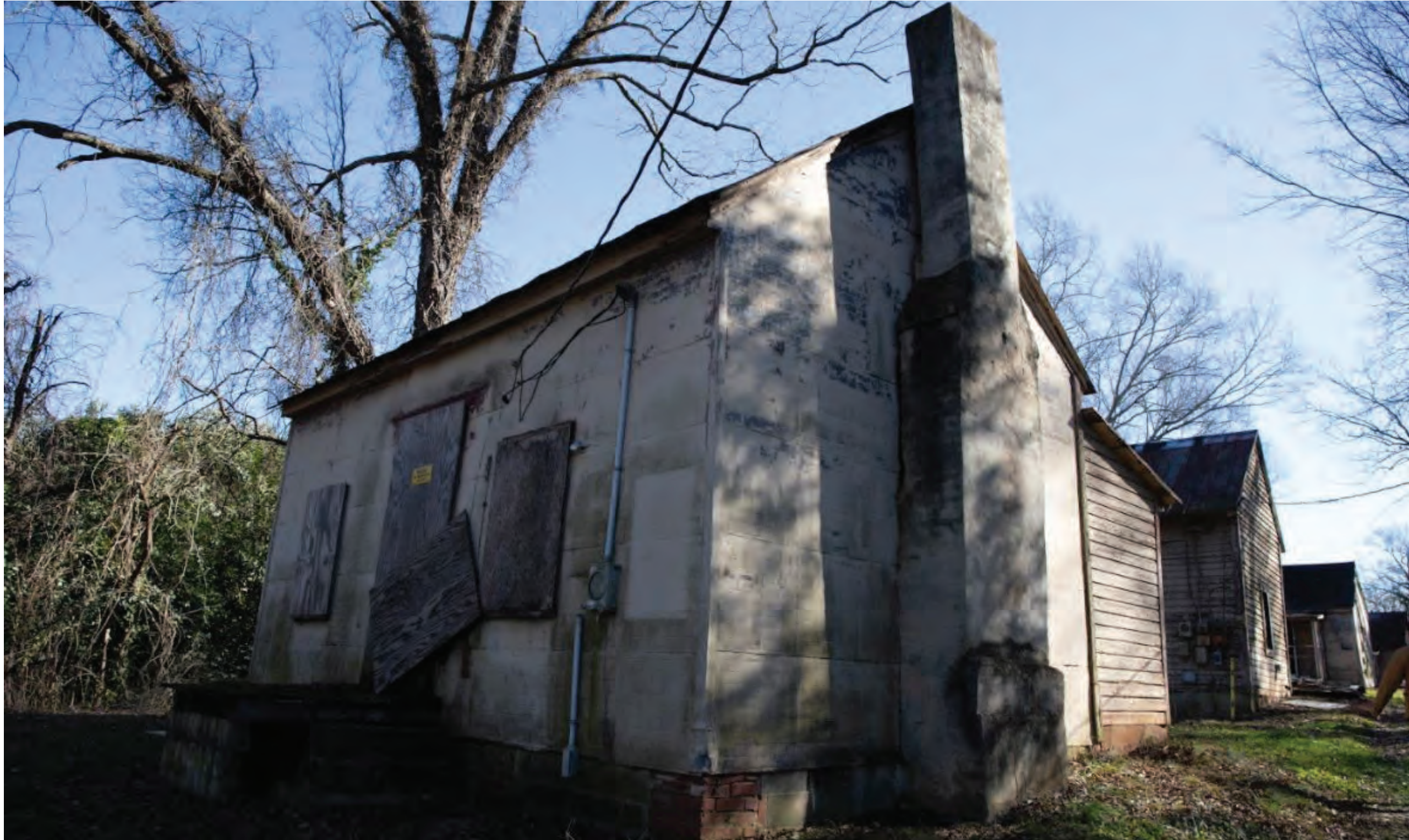
312 East Morris Street north elevation
