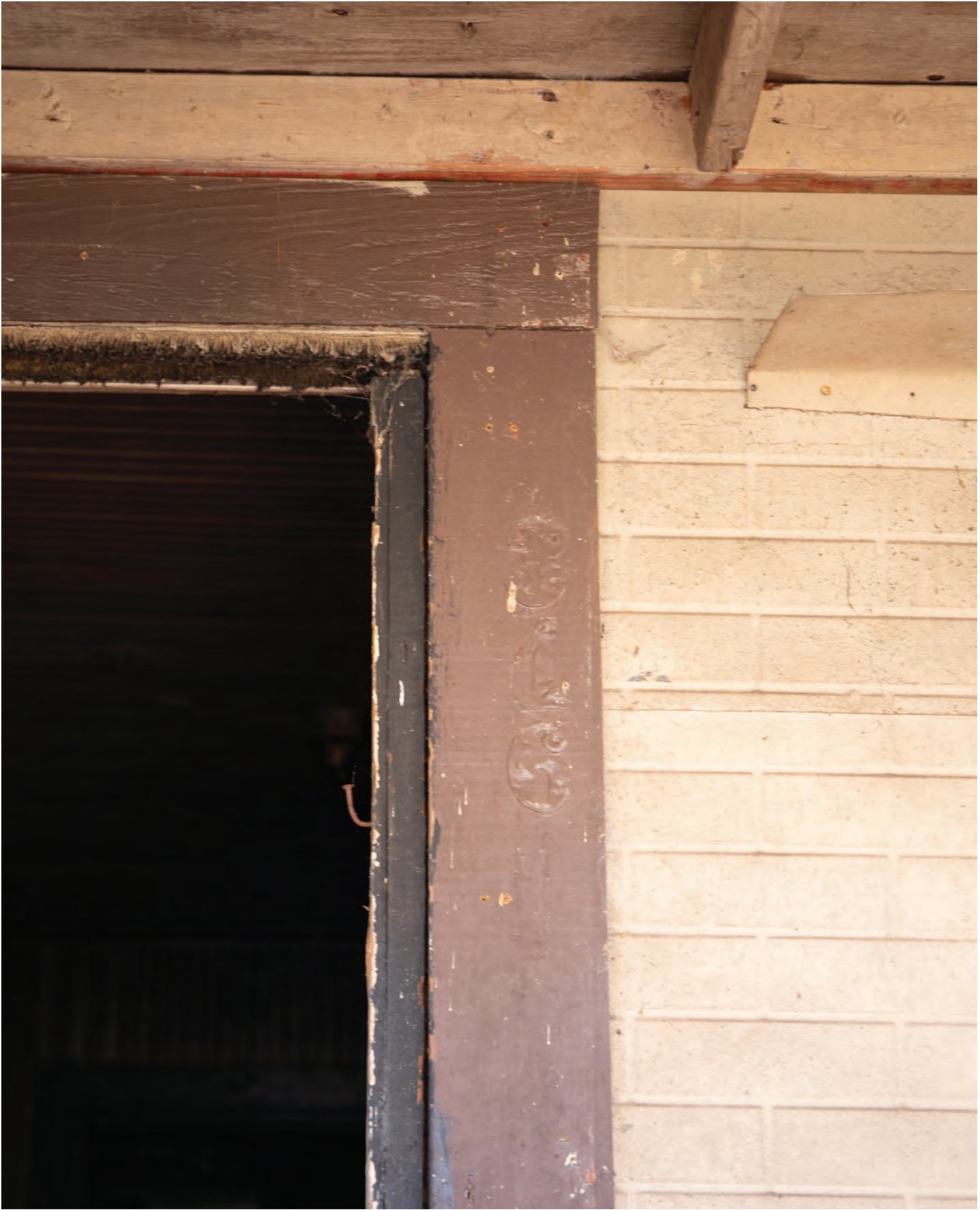
Door opening and surround
