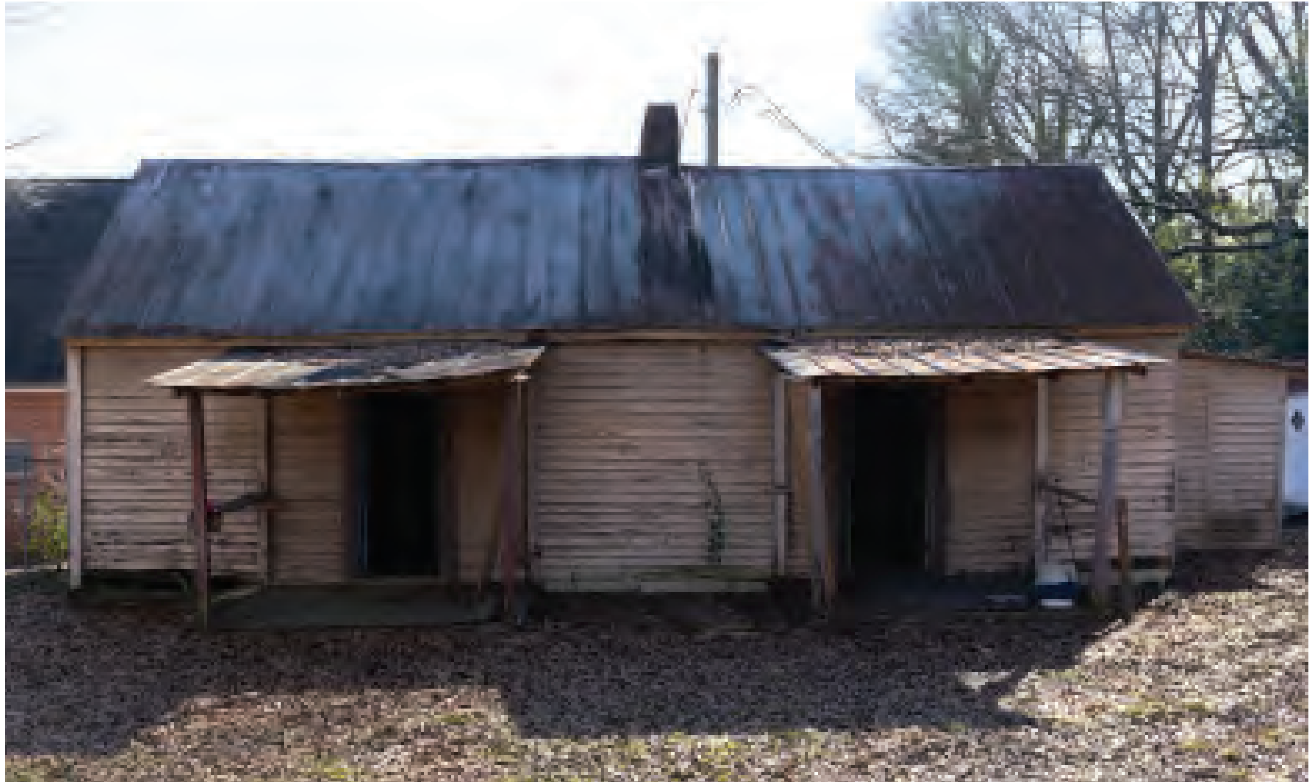
318 East Morris Street north elevation
